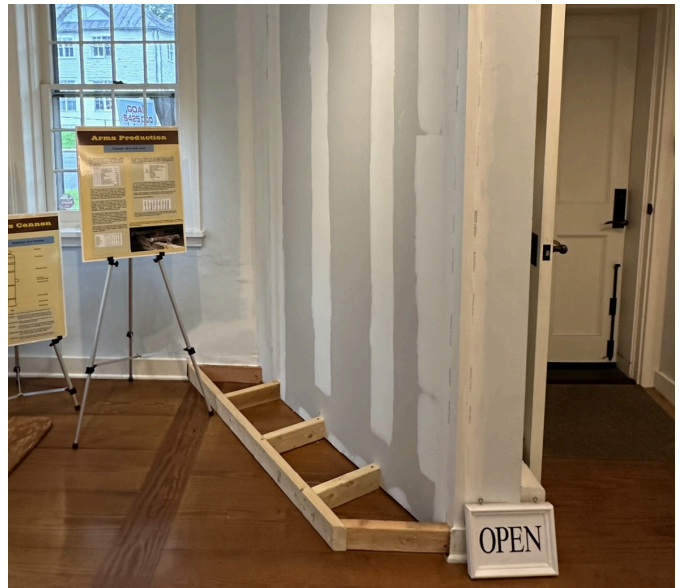
Academy Building work in process
