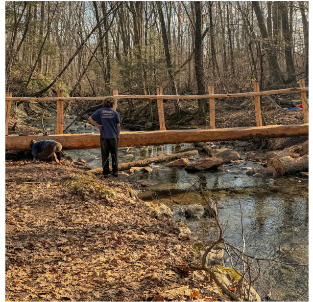
Working with SALT, Greenagers built a bridge from a fallen tree on Yoakum Preserve.
