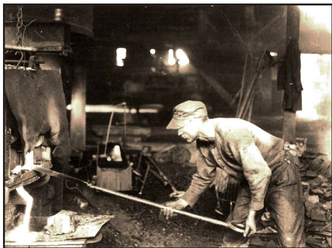
Puddler at work refining pig iron
