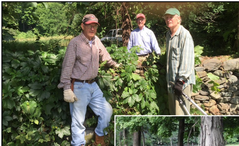
Clearing vegetation from wall. Left to right: Tom Key, John Arnold, George Massey
