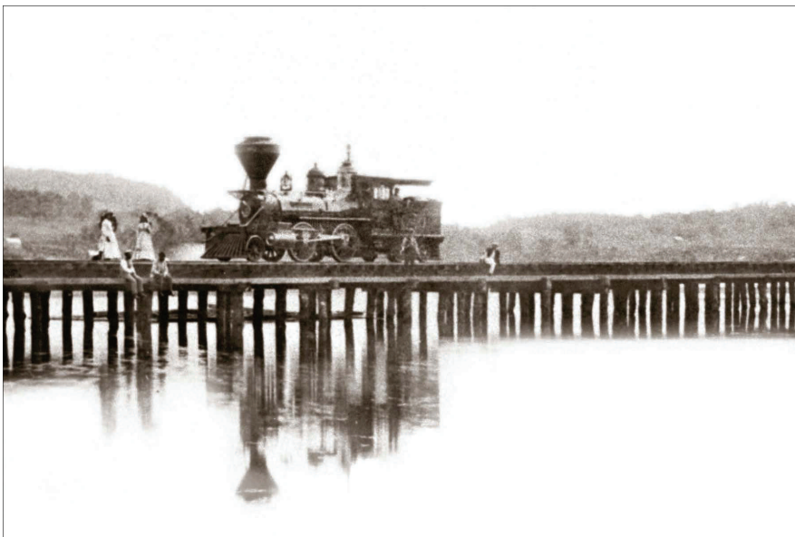
Steam engine on the Twin Lakes trestle (Salisbury Association archives)
